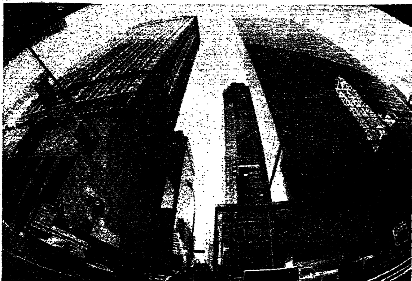
Side by side in New York—Philip Johnson's post-modern AT&T headquarters (left) is flanked by orthodox modern IBM headquarters, both recently completed
